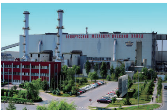
BMZ Steel Work
