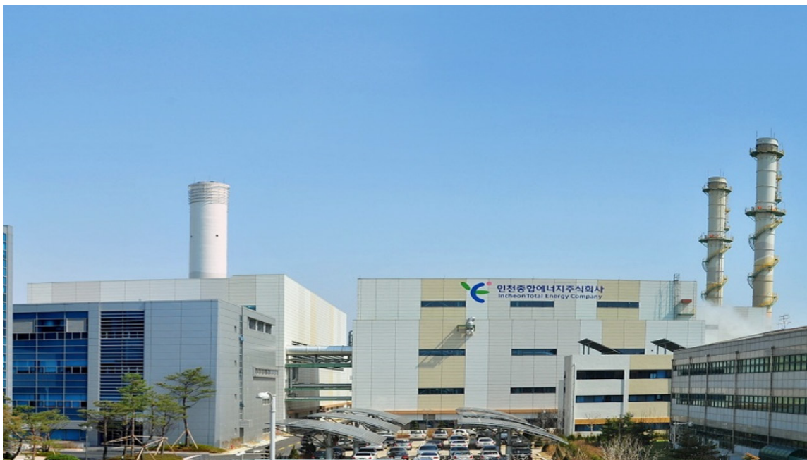
Campus of Incheon Total Energy 仁川综合能源都厂区
