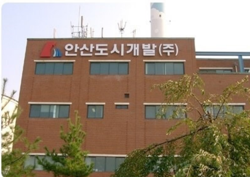
Ansan District Heating Company 安山都市开发
