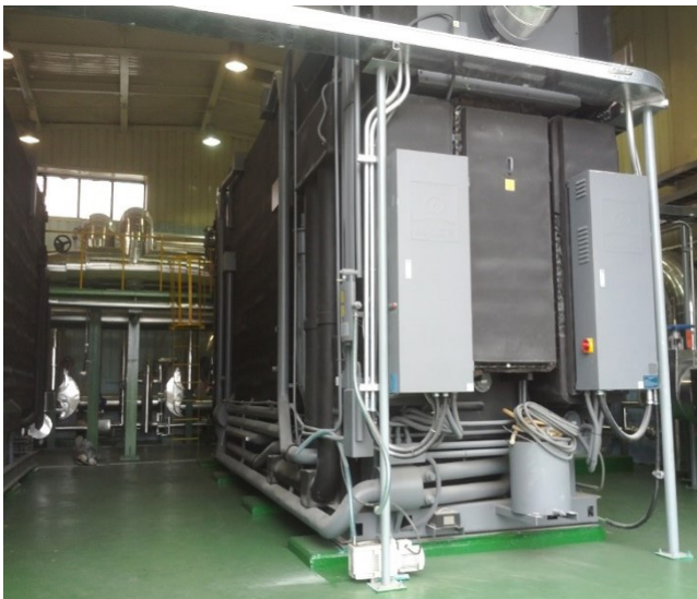
Machine room of Ilsan Power Plant heat pump 日山电厂热泵机房
