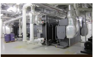
Heart of CCHP, Absorption Chiller 冷热电联产的心脏,吸收式空调
